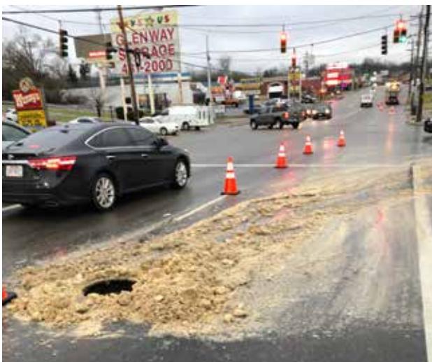
Grease blockage in sewer on Glenway Avenue caused traffic disruptions in Dec. 2019. The grease was improperly discharged to the sewer by a restaurant. The restaurant was fined for improper disposal. Cost recovery fines were also issued.
